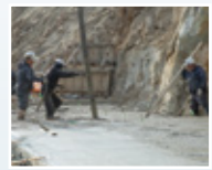
Large work area
