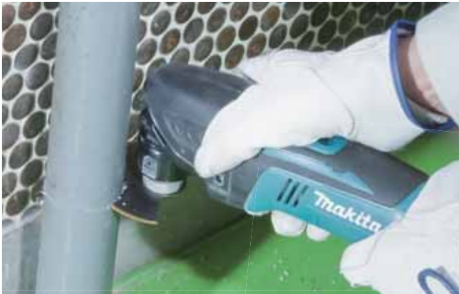
Cutting PVC, FRP pipes
