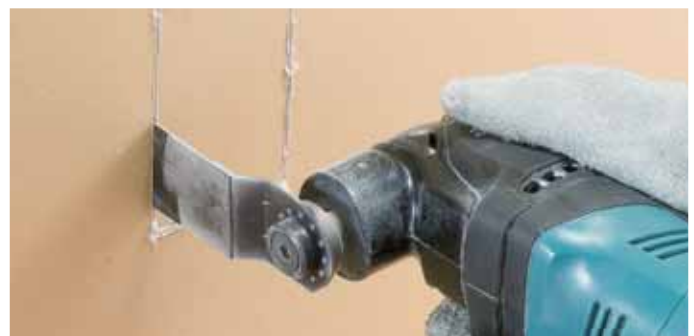
Cutting plasterboards
