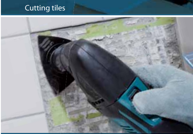
Removing mortar, tile adhesive
