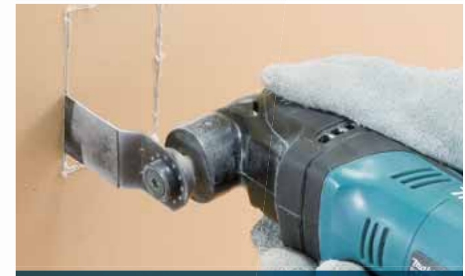
Cutting plasterboards
