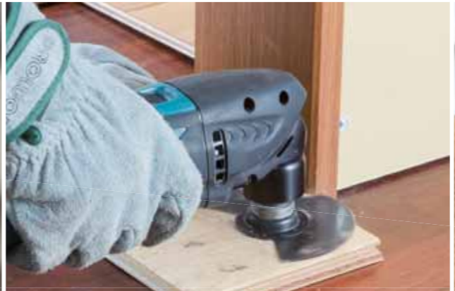
Wood flush cutting
