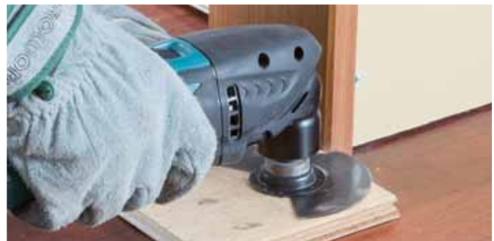
Wood flush cutting
