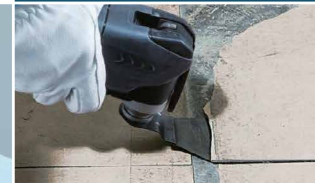
Scraping floor tiles
