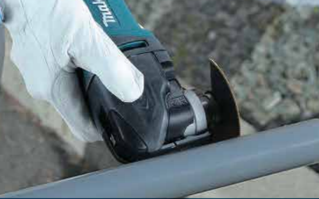
Cutting PVC, FRP pipes
