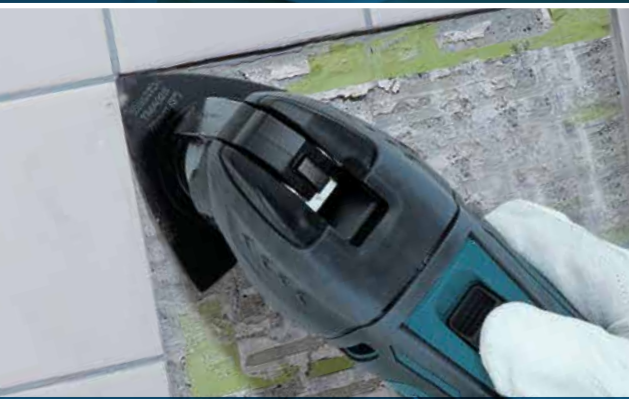
Removing mortar, tile adhesive
