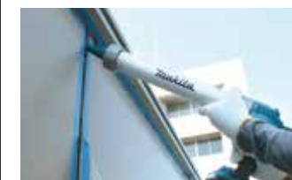
For Sealing work with two-component system
