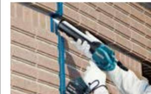
For Bonding of external wall, window frame.
