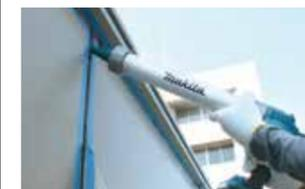
For Sealing work with two-component system
